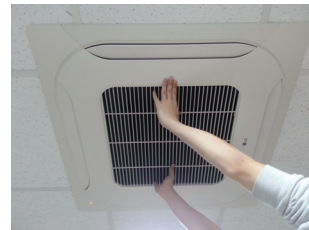
Check the left, right and central sections
